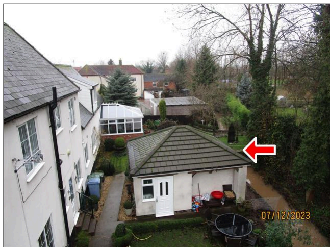
26.3 Item 1(Picture) Roof to summerhouse
