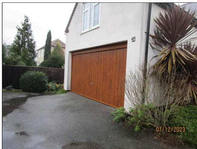
25.0 Item 1(Picture) Garage vehicle access door
