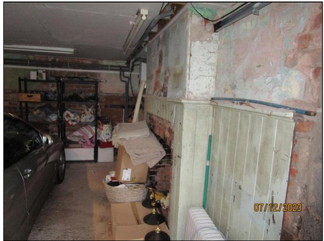
25.3 Item 2(Picture) Internal of the garage
