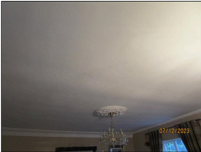
17.3 Item 1(Picture) Ceilings of likely timber lath
