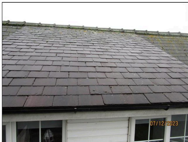
10.3 Item 4(Picture) Roof to dormer
