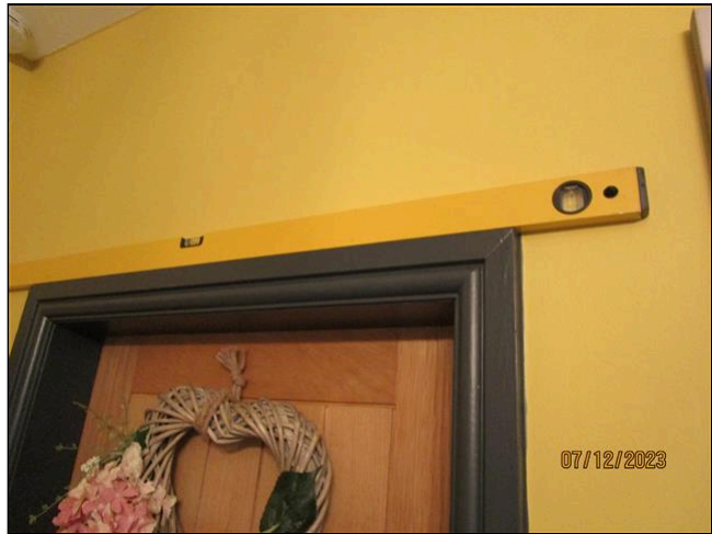
22.3 Item 2(Picture) Door level checks
