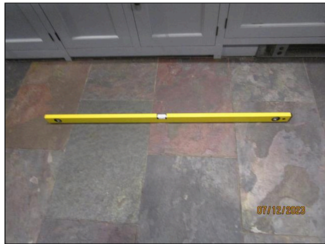
3.3 Item 4(Picture) Movement checks to floors
