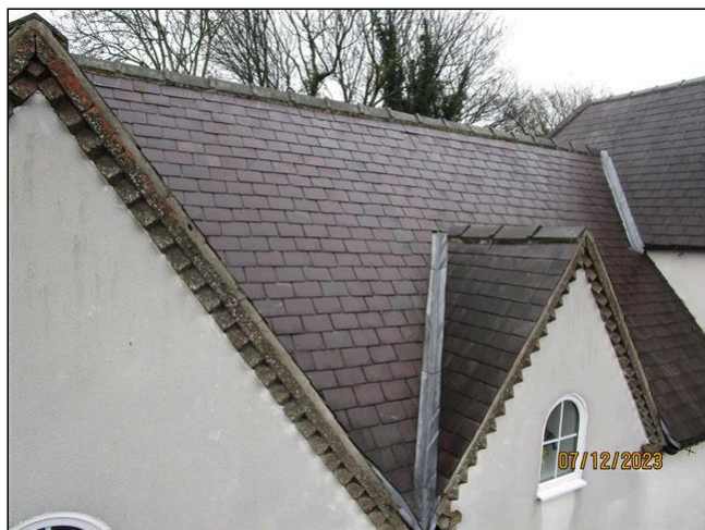
10.3 Item 1(Picture) Front roof
