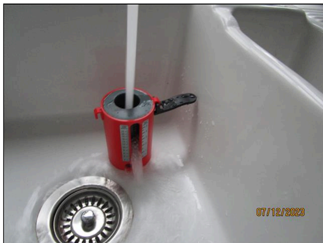
30.0 Item 1(Picture) Water flow checks
