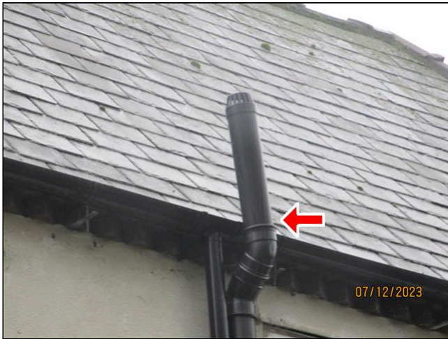
12.3 Item 1(Picture) Soil vent pipe at the rear
