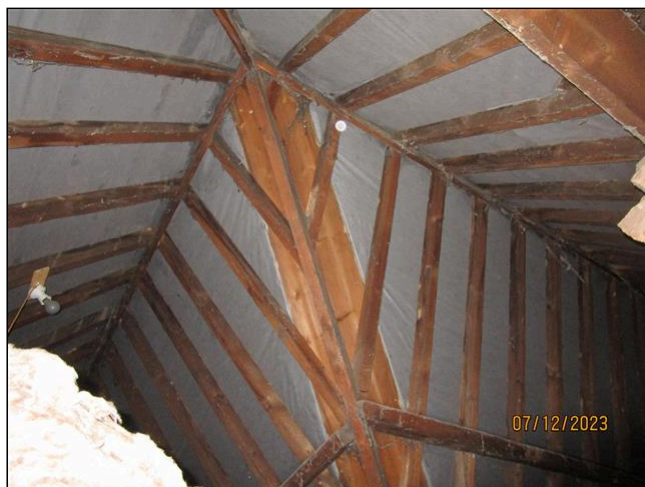
16.0 Item 2(Picture) Roof construction
