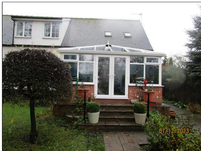
15.0 Item 1(Picture) Conservatory at the rear
