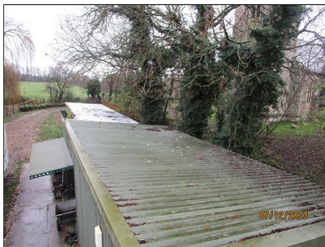
26.3 Item 4(Picture) Garage metal roof
