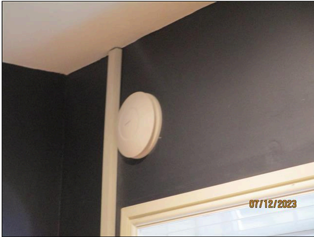
24.1 Item 1(Picture) Kitchen vent near window
