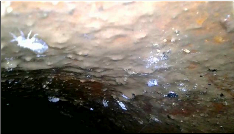
32.3 Item 4(Picture) Drain camera small sewer
