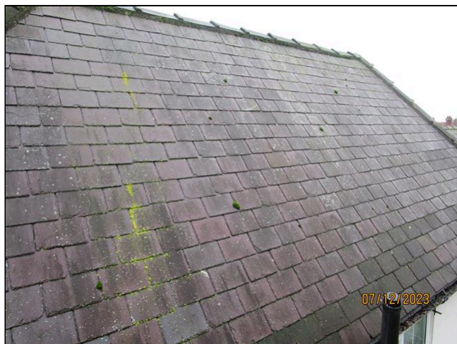
10.3 Item 3(Picture) Rear roof
