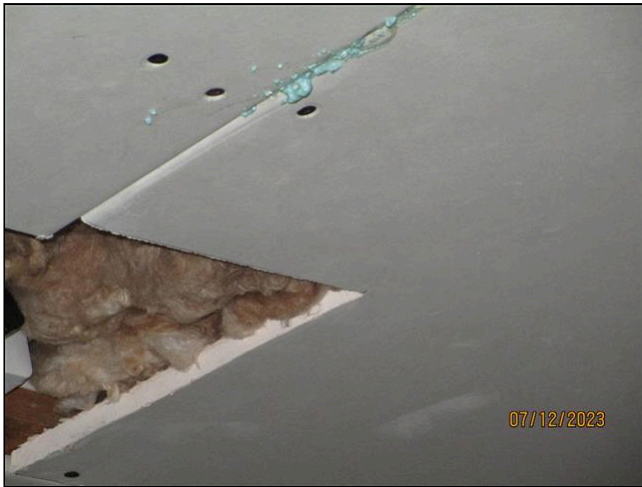
25.3 Item 1(Picture) Garage ceiling insulated
