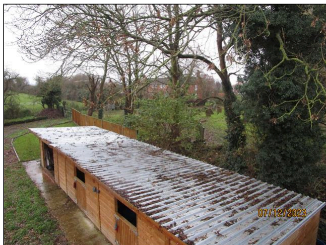
26.3 Item 7(Picture) Metal roof to the Equestrian Buildings
