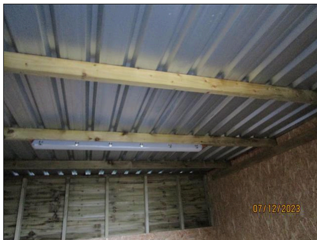
26.3 Item 8(Picture) Internal roof to Equestrian Buildings
