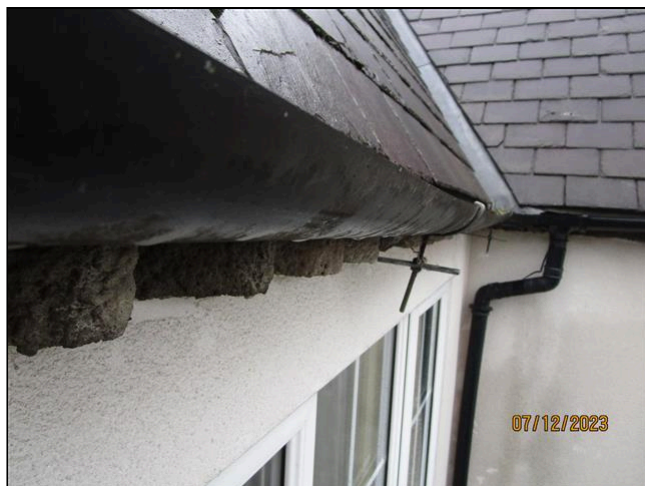
11.3 Item 1(Picture) Gutter fittings and downpipe
