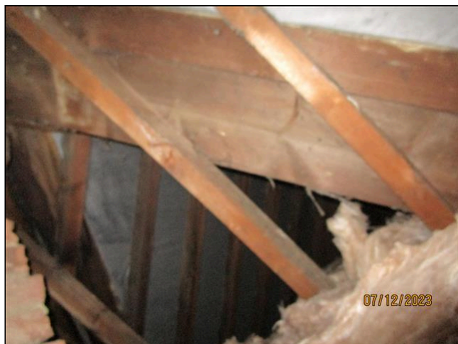
16.3 Item 1(Picture) Roof timbers
