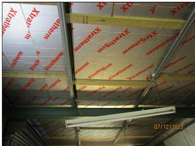
26.3 Item 5(Picture) Garage roof insulation
