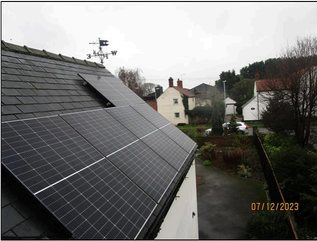
10.3 Item 5(Picture) Roof to the Left side
