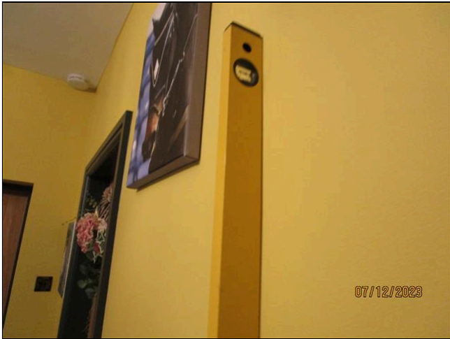
3.3 Item 5(Picture) Internal movement checks
