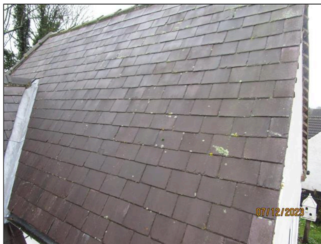
10.3 Item 2(Picture) Front roof
