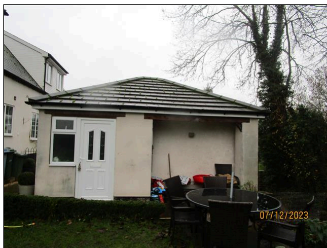
26.0 Item 1(Picture) Summerhouse at the rear
