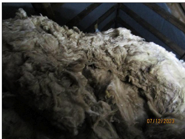
16.3 Item 3(Picture) Insulation
