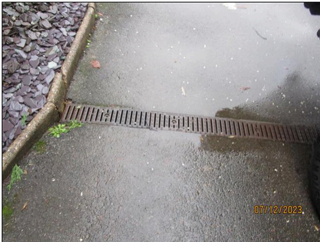
32.0 Item 3(Picture) Channel drain on driveway
