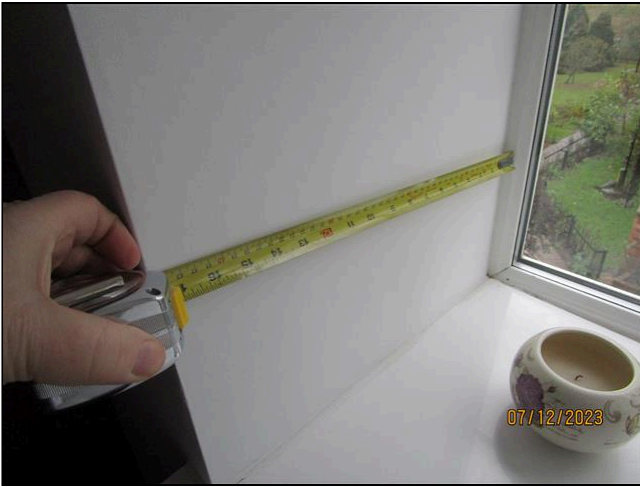
18.3 Item 3(Picture) Checks for wall insulation
