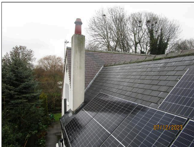
9.0 Item 2(Picture) Brick chimney with cement render
