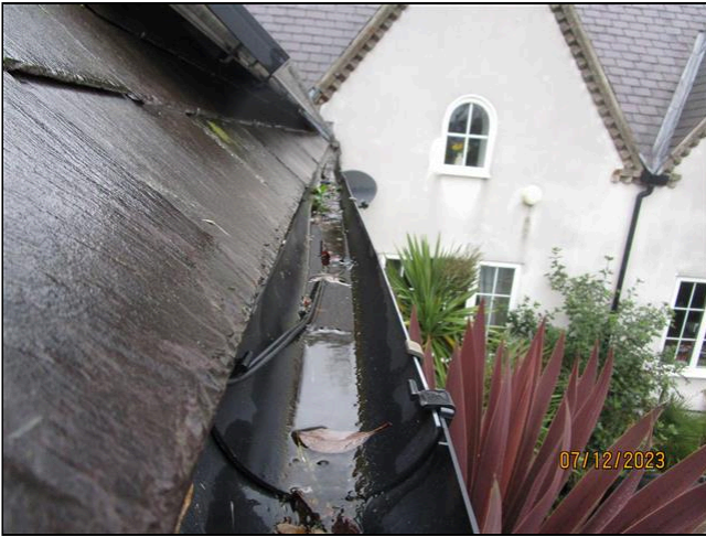
11.3 Item 3(Picture) Guttering
