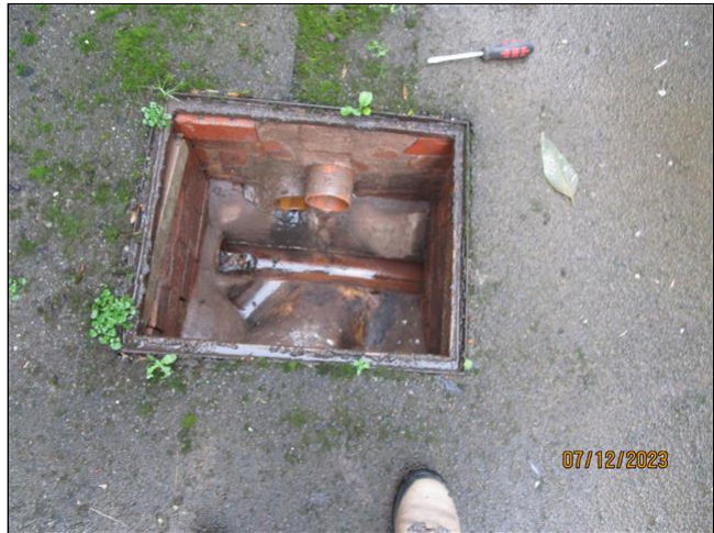
32.0 Item 2(Picture) Drain construction
