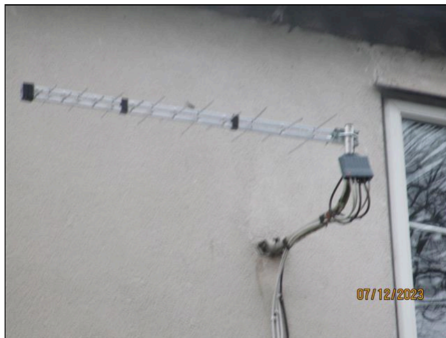
33.0 Item 2(Picture) Aerial at the rear
