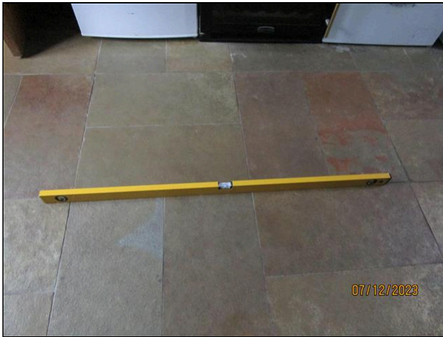
19.3 Item 1(Picture) Floor level checks
