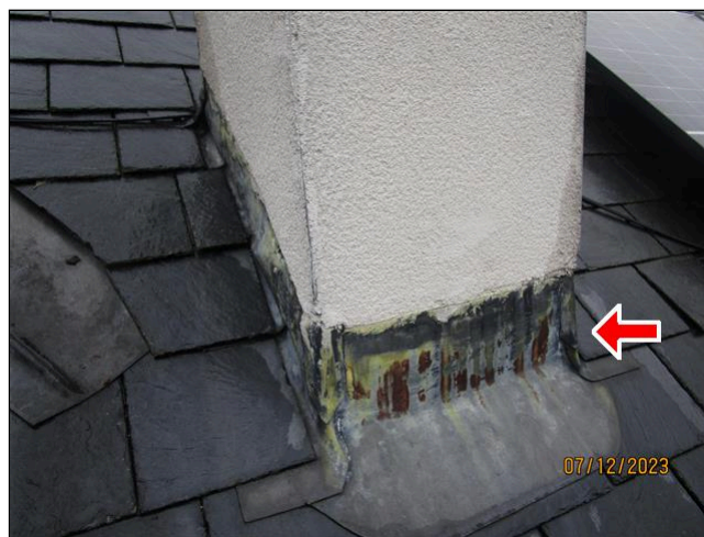
9.3 Item 2(Picture) Lead flashing at the base
