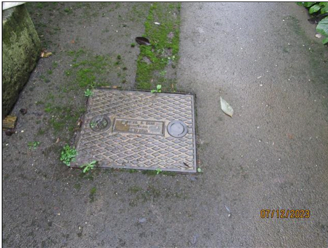
32.0 Item 1(Picture) Drain cover at the side of the property
