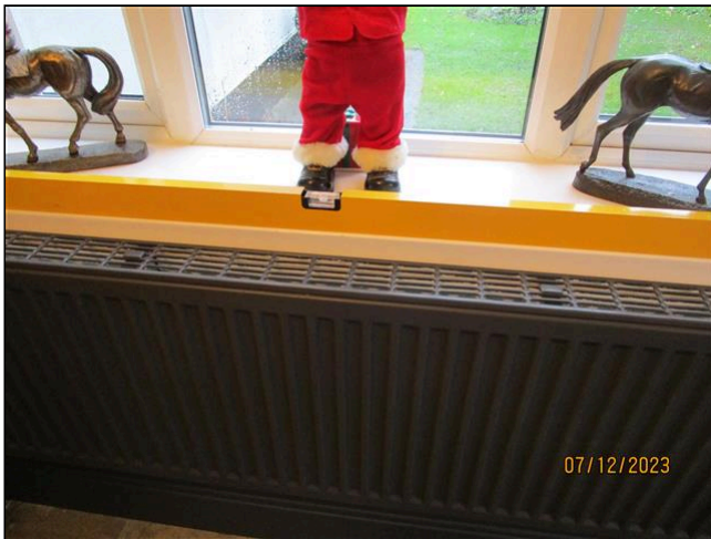
14.3 Item 3(Picture) Window level checks
